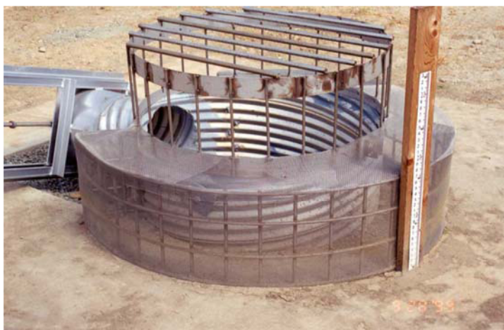
Figure 1 Example of Extended Detention Outlet Structure
