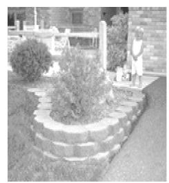
A **Gravity** retaining wall system depends on its weight and geometry to counteract the lateral earth pressure and other lateral forces. These walls generally utilize modular concrete units in a running bond without the use of mortar.
