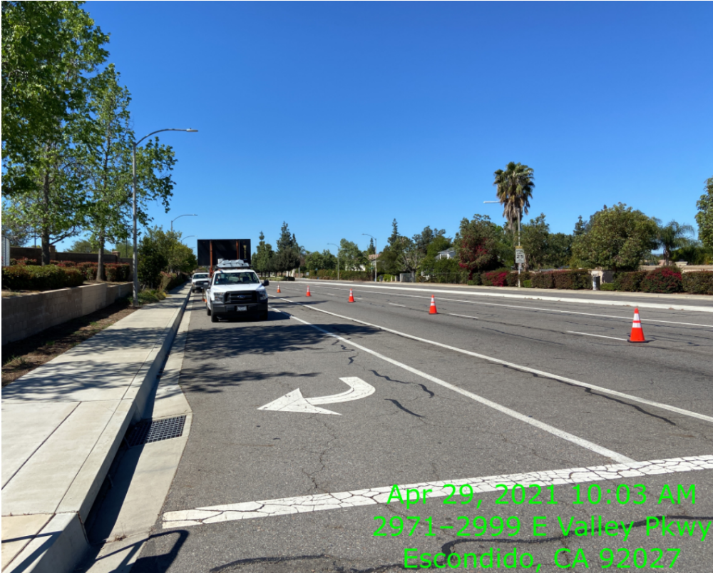
Figure 1 – Street Light installation
