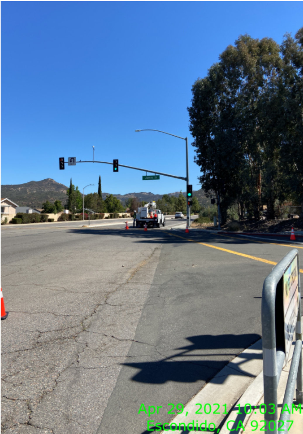
Figure 3 – Safety Light Installation
