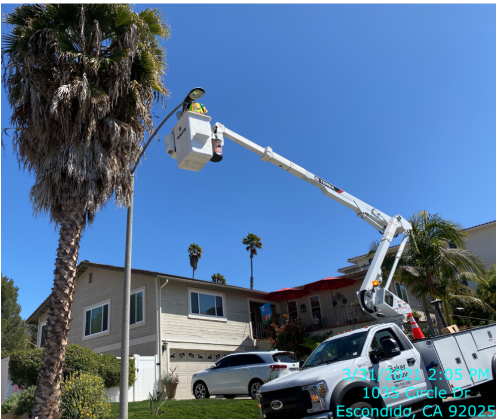
Figure 2 – Street Light installation
