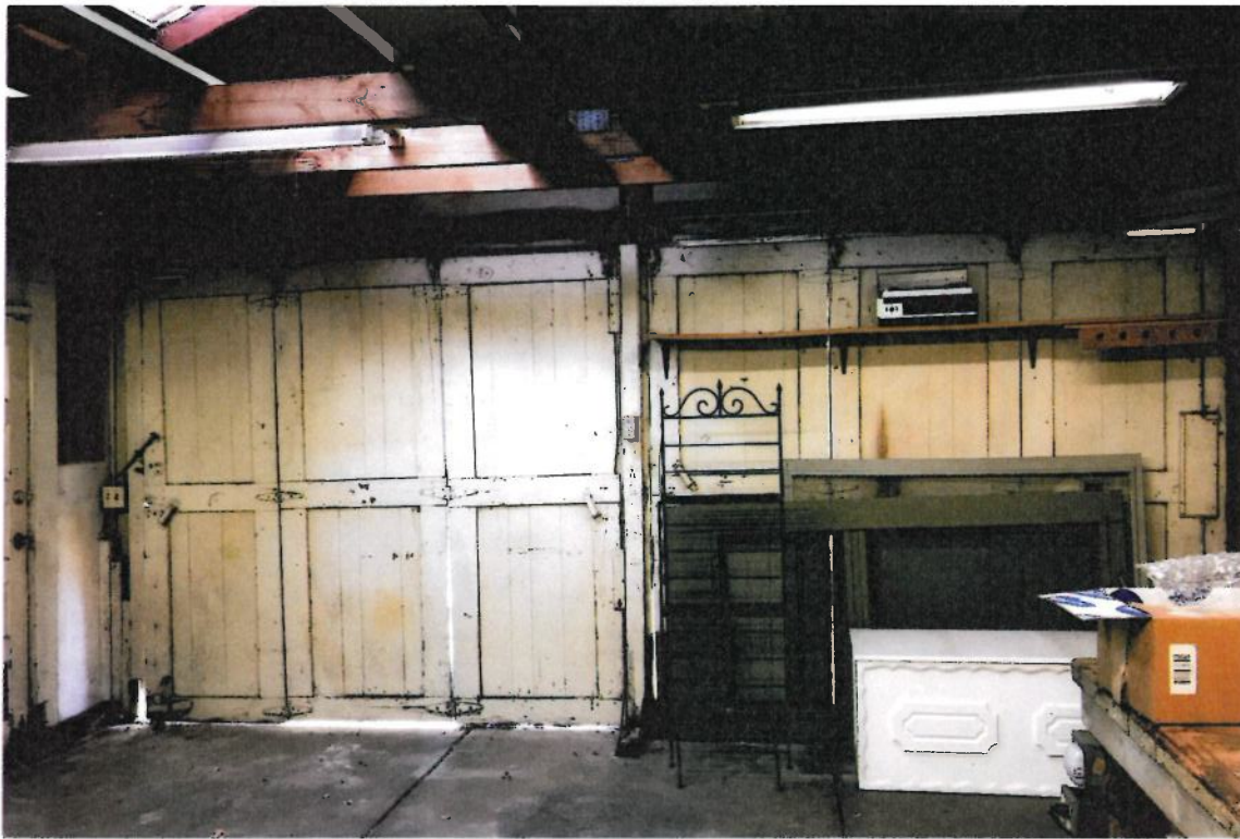
South facing Garage Interior
