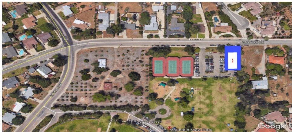
Proposed location for Mountain View Park pump station
