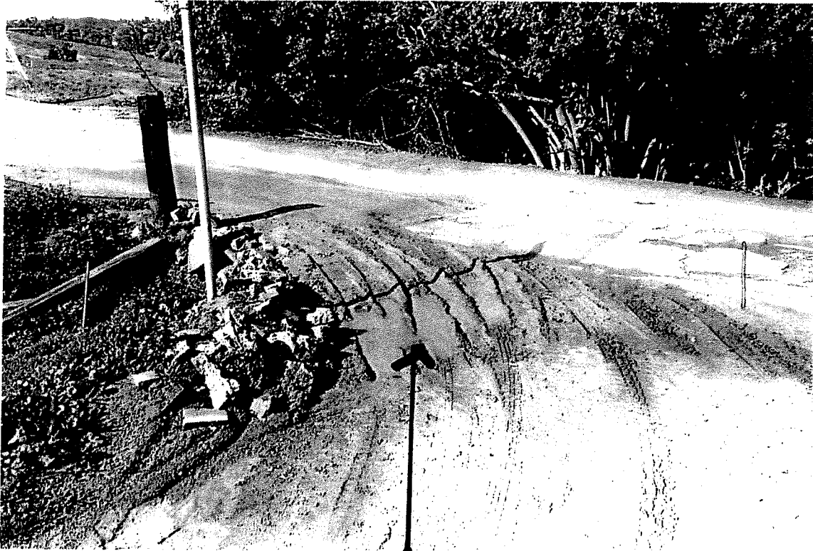
MUD RUNOFF DUE TO PART CLOGGED DRAIN
