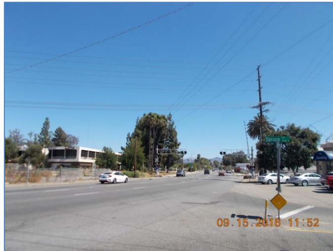
Figure 2. Intersection at Spruce Street and Grand Avenue (ESC_134) with significant wire crossings overhead. Photo taken from the south side of the intersection looking west.
