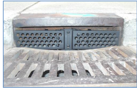
Figure 9. Powder Coated Automatic Retractable Screen
