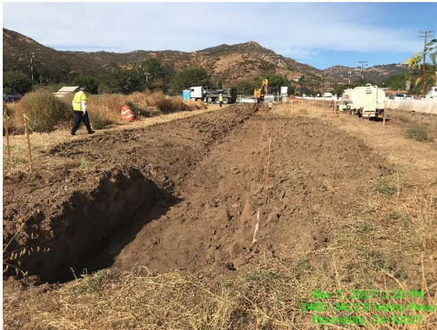
Grading Excavation for Bio Filtration Basin
