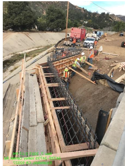
Forming and Rebar Installation for Bridge Abutment and Wing Wall
