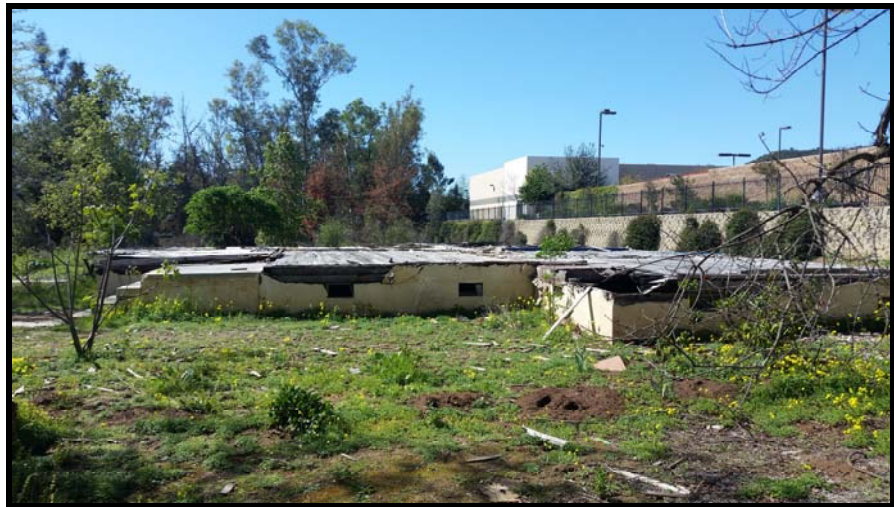
Photograph 4: View of existing building footing from former structures, facing north.
