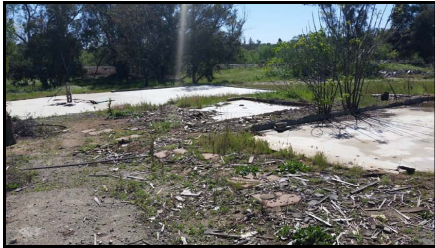
Photograph 5: View of existing building footings from former structures, facing northeast.
