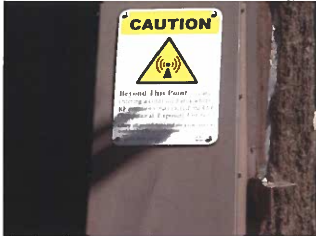
Caution sign at monopole
