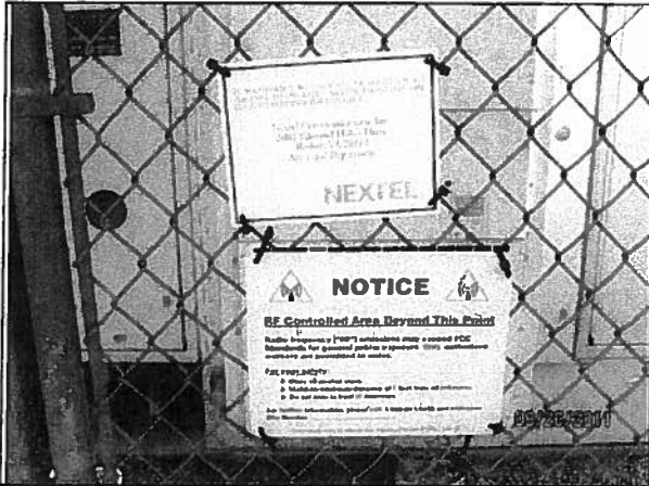
13. Detail of signage on Nextel enclosure.
