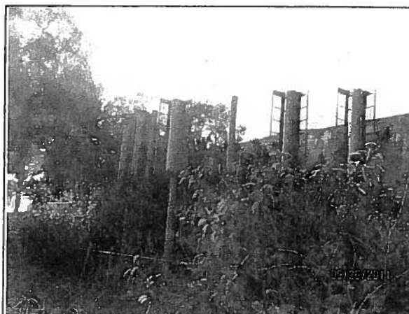
10. View west-northwest toward Nextel sector A and B antennas.
