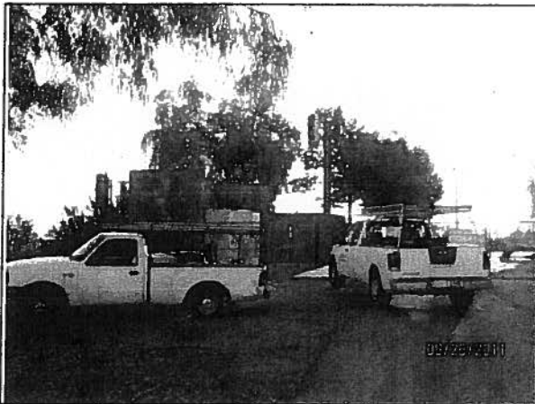
1. View west-southwest; overview of Sprint and AT&T facilities.
