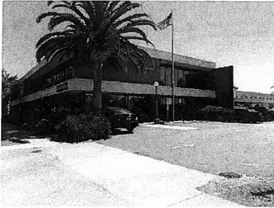
View of the office building looking east from the western portion of Sub-Area C
