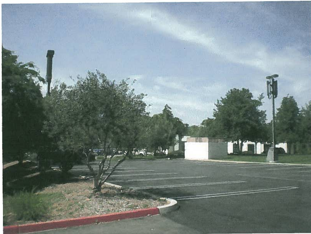
Figure 11: T-Mobile's Monopoles Overview
