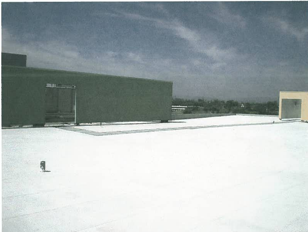
Figure 9: Main Overview facing North West
