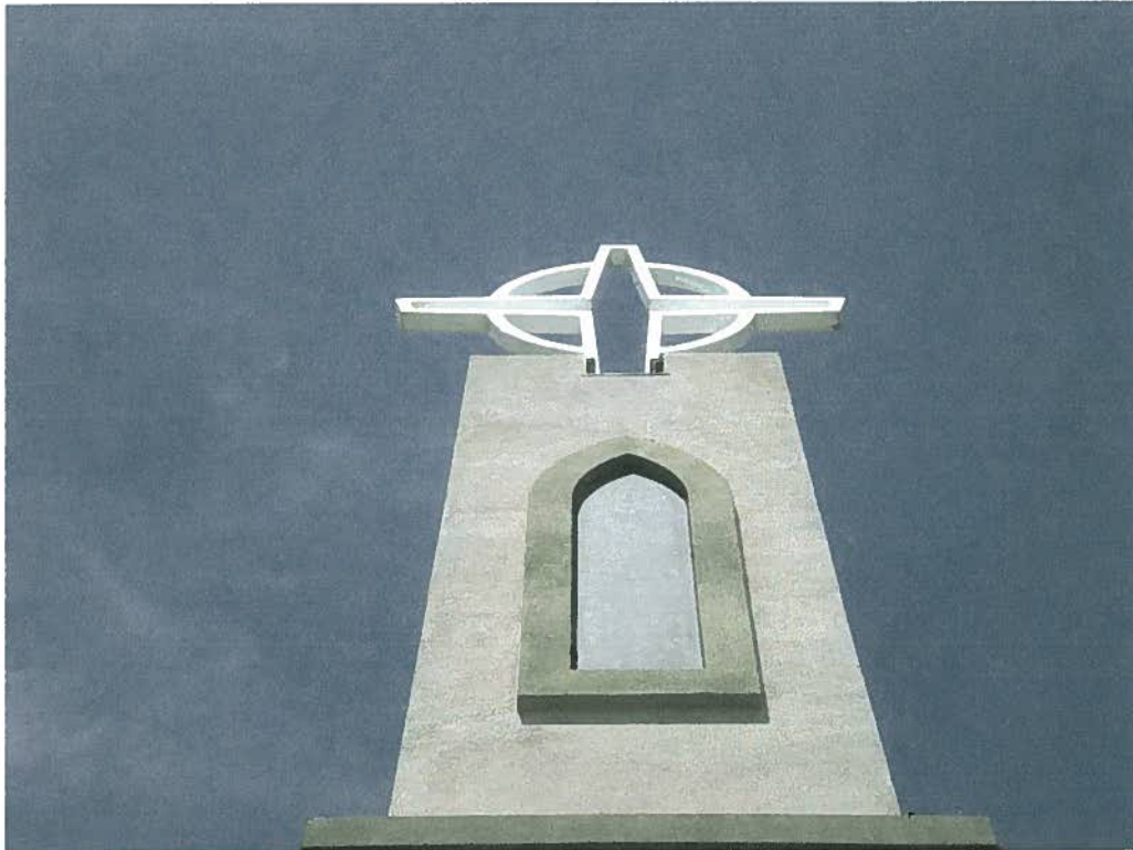
Figure 8: AT&T Mobilify, LLC Antennas #21 and #22 Location
