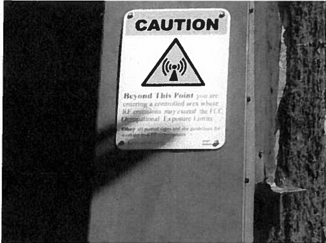
Caution sign at monopole
