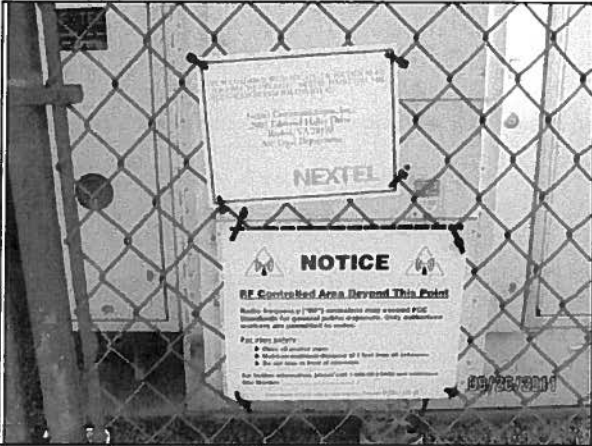
13. Detail of signage on Nextel enclosure.
