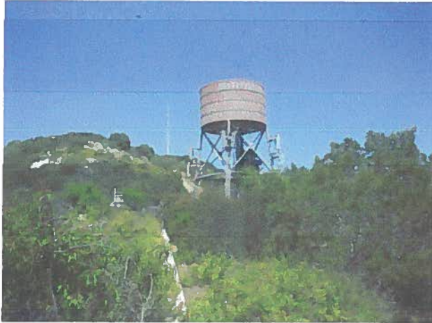
Faux water tank General View
