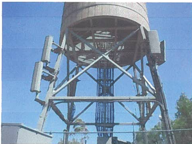
Nextel Sector A (2 left), Verizon Sector B & C (2 right)
