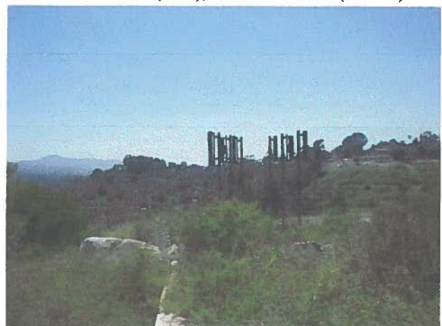
Sprint/Clearwire All Antennas (6 total)
