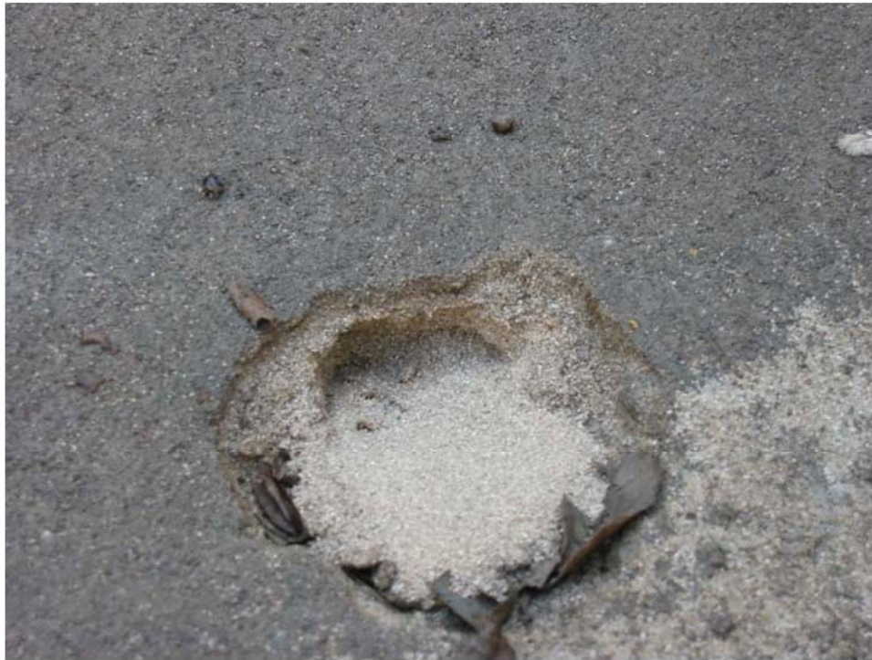
Figure 7 Formation of Clogging Crust on Filter Bed
