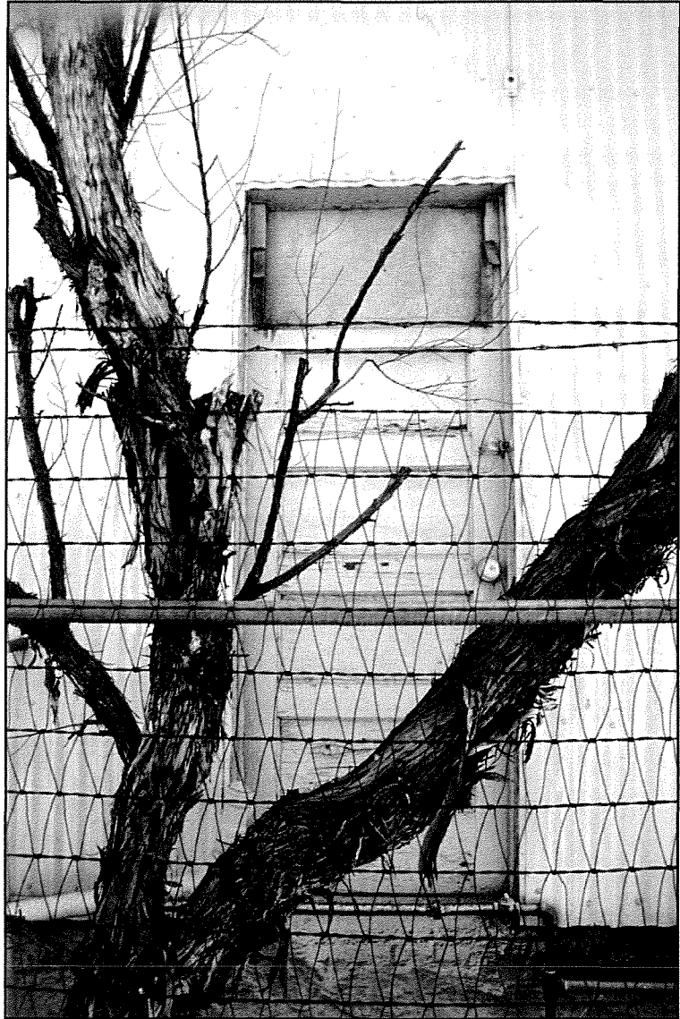
PHOTOGRAPH 15 Entrance Door in North Wall
