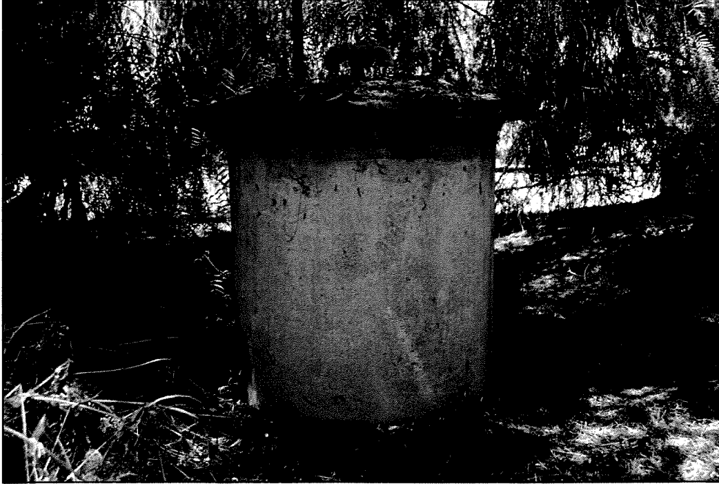
PHOTOGRAPH 26 Concrete Pipe with Concrete Cap Located Next to Loading Dock
