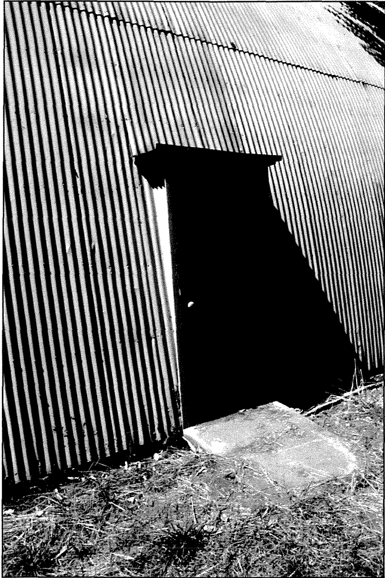
PHOTOGRAPH 12 Entrance Door in East Wall
