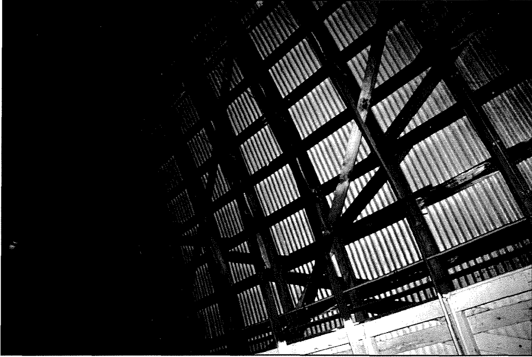
PHOTOGRAPH 16 Wooden Truss Structure of EMWD Shop/Warehouse
