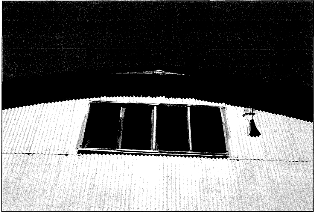
PHOTOGRAPH 9 Hopper Windows at Apex of South Wall
