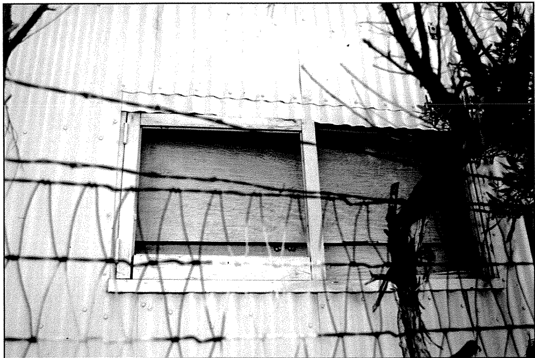
PHOTOGRAPH 14 Detail of Windows in North Wall
