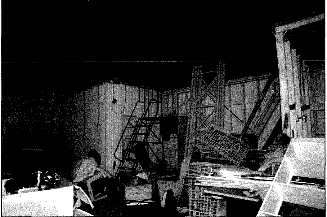
PHOTOGRAPH 23 Small Enclosed Room on East Side of Wall Dividing Third and Fourth (Southern) Spaces
