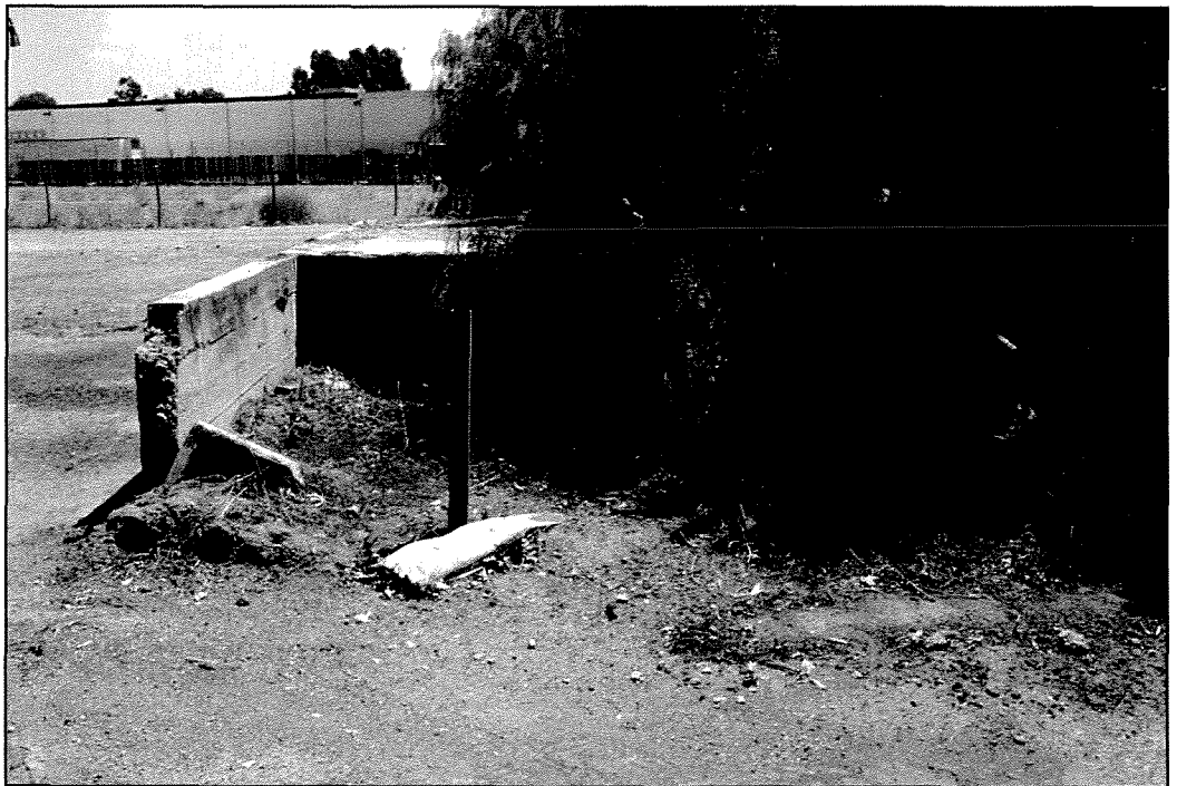
PHOTOGRAPH 25 Open End of Loading Dock with Ramp on Right Side
