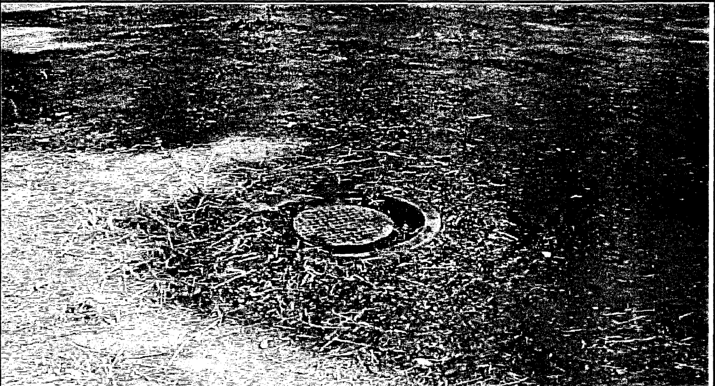
View of blue metal cover southeast of the building that might be for valving or a water UST.
