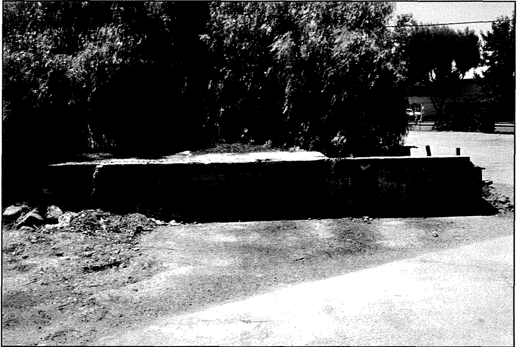
PHOTOGRAPH 24 Loading Dock in Yard Looking West
