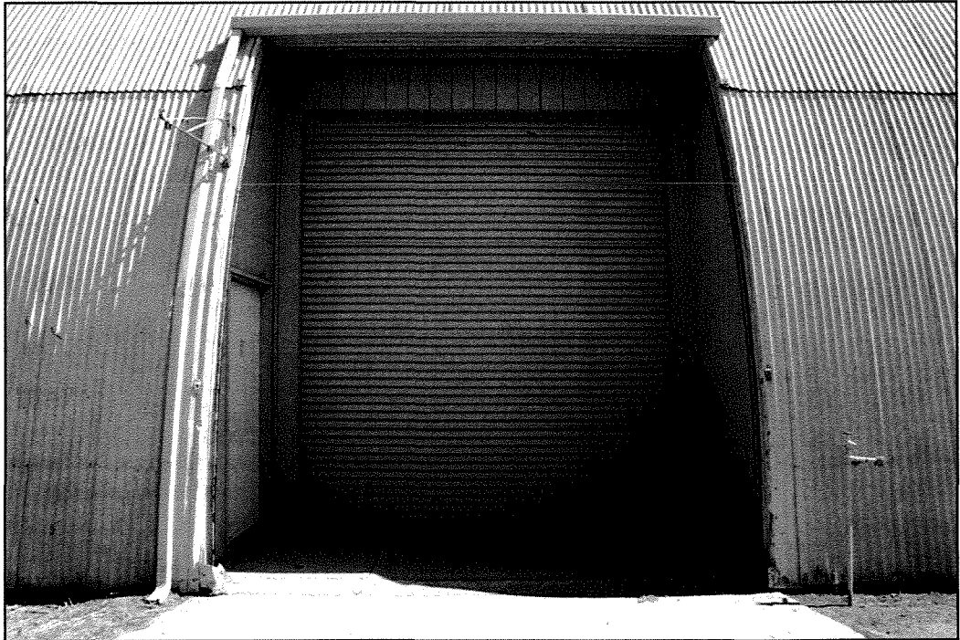
PHOTOGRAPH 4 Example of Mounting of Northern 3 Roll-Up Doors
