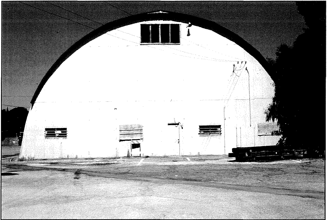
PHOTOGRAPH 7 South Elevation of EMWD Building
