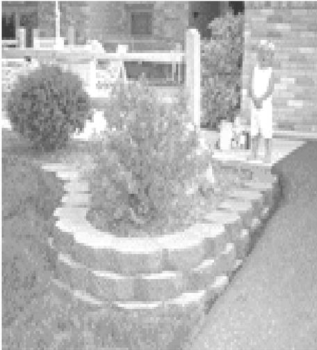
A **Gravity** retaining wall system depends on its weight and geometry to counteract the lateral earth pressure and other lateral forces. These walls generally utilize modular concrete units in a running bond without the use of mortar.
