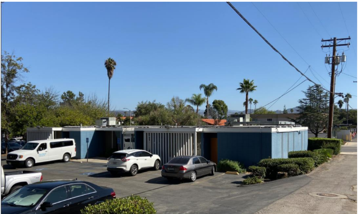
West Façade / Parking Lot
