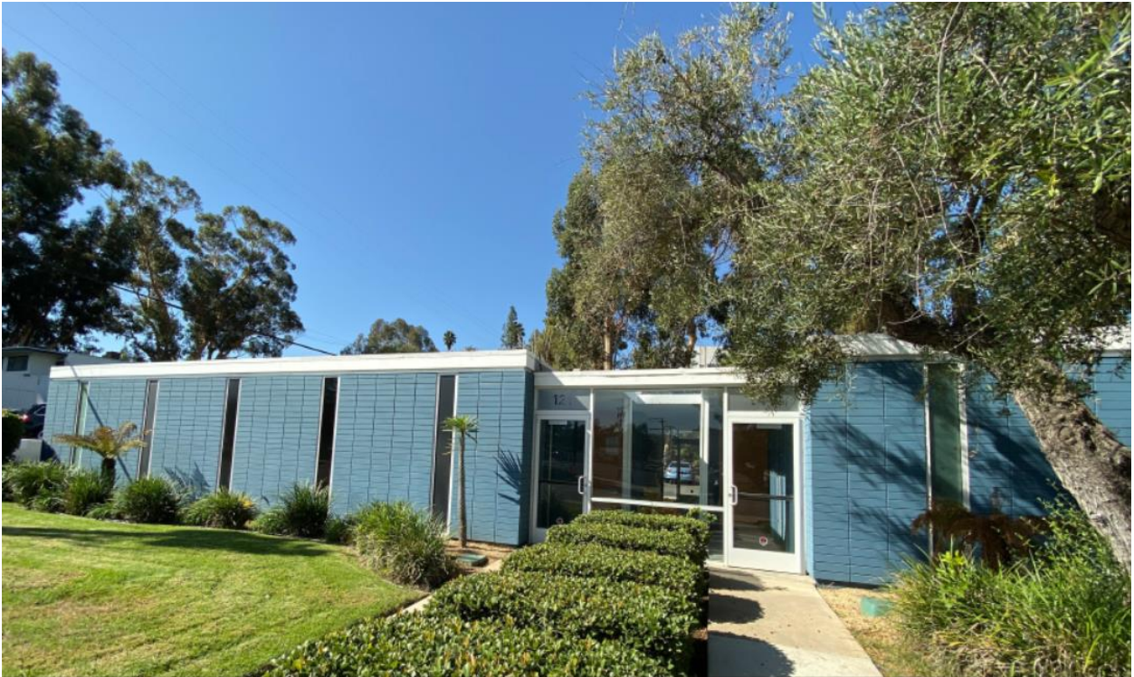
East Façade / Building Entrance
