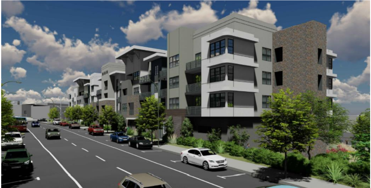
Senior Apartments (one building)
