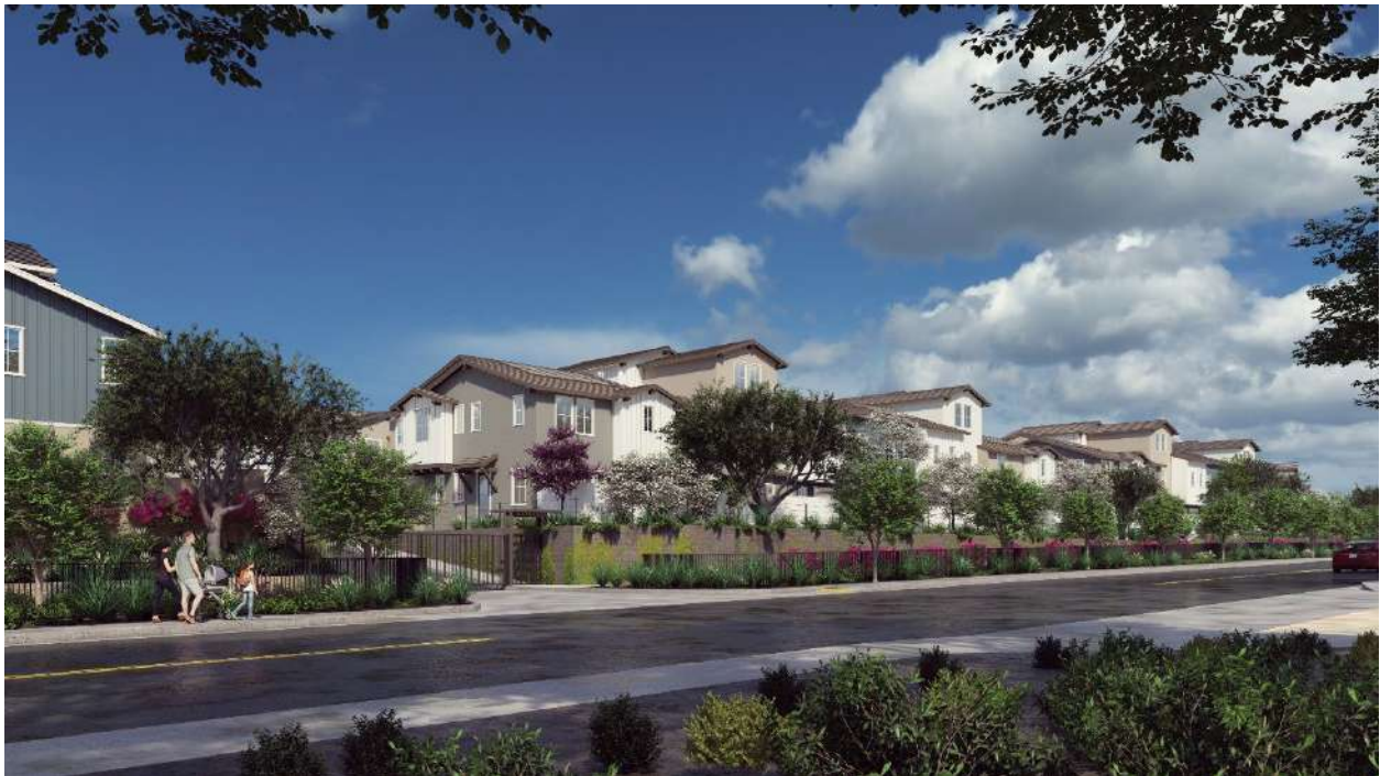
Looking west and northwest along Iris Lane towards secondary gated access
