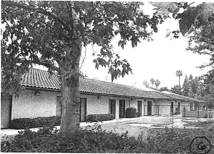
Looking along southeastern building elevation
