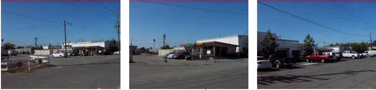
Typical aging, underutilized industrial properties along W. 4 th Avenue in the Mercado area.
