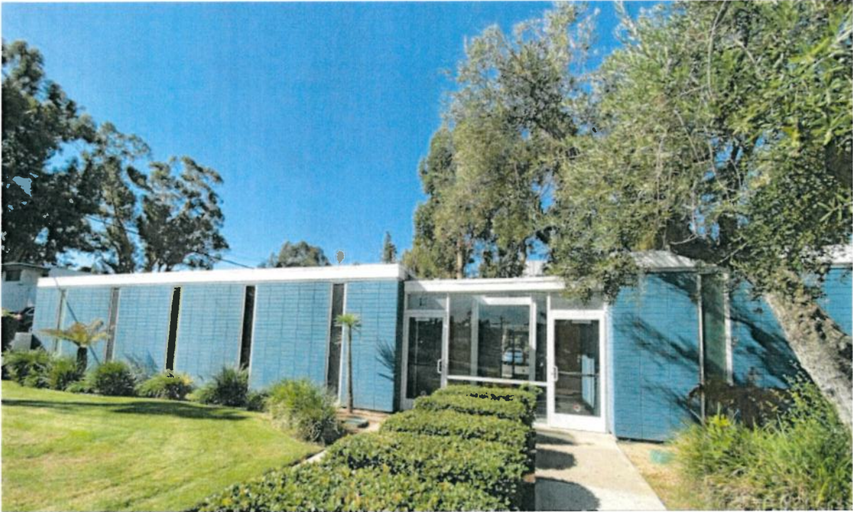
East Façade / Building Entrance
