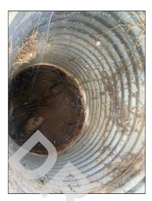
Photo 11: Interior of a drainage/irrigation pipe from former onsite structures.
