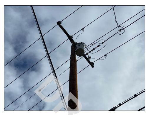
Photo 15: Pole-mounted transformer.
