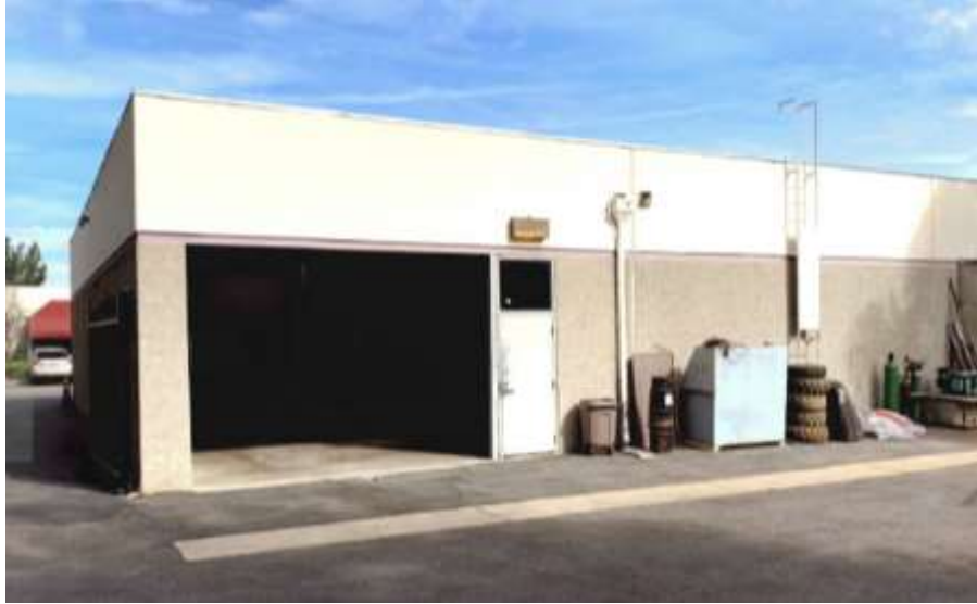
UNIT 1 BUILDING REAR
