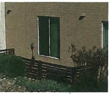
1. WOOD OR VINYL FENCE TO SCREEN MECHANICAL UNITS NOTE: WOOD A/C SCREENS TO BE "EARTH TONE" COLORS TO MATCH THE RESIDENCES WOOD/VINYL SCREEN FENCE DETAIL
