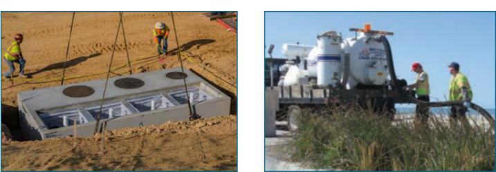
The Modular Wetlands<sup>®</sup> is simple, easy to install, and has a space-efficient design that offers lower excavation and installation costs compared to traditional tree-box type systems. The structure of the system resembles precast catch basin or utility vaults and is installed in a similar fashion.
