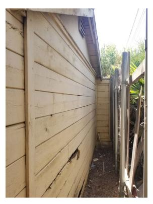
Plate 42. South façade with side gabled roof and double-vee rustic wood siding, looking east. An attached lean-to clad in wood siding is extant on the east end. This addition was added to the original duplex. Photo taken on July 9, 2020.
