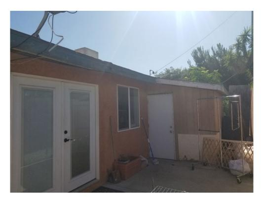
Plate 51. South façade with stucco clad enclosed breezeway addition and French doors, looking southeast. Notice the vertical wood boards that clad the original 1947 portion.
