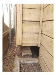
Plate 43. Post on concrete pier foundation on south façade, looking west. Photo taken on July 9, 2020.
