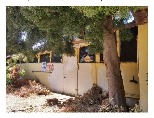
Plate 39. North façade of east addition with shed style roof and fixed clerestory windows, looking southwest. Photo taken on July 9, 2020.
