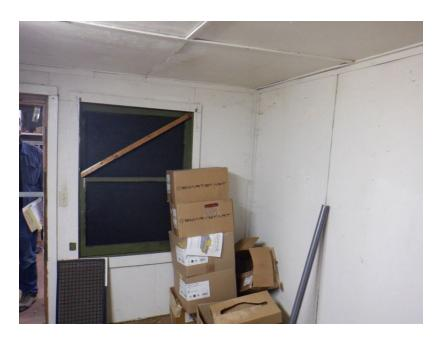
Plate 44. Interior of addition on the south façade, looking north. Notice the original exterior wood window frame that was enclosed when this addition was added, looking north.
