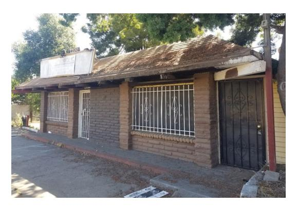
Plate 34. West façade with adobe brick veneer and faux rafters, looking northeast. Photo taken on July 9, 2020.
