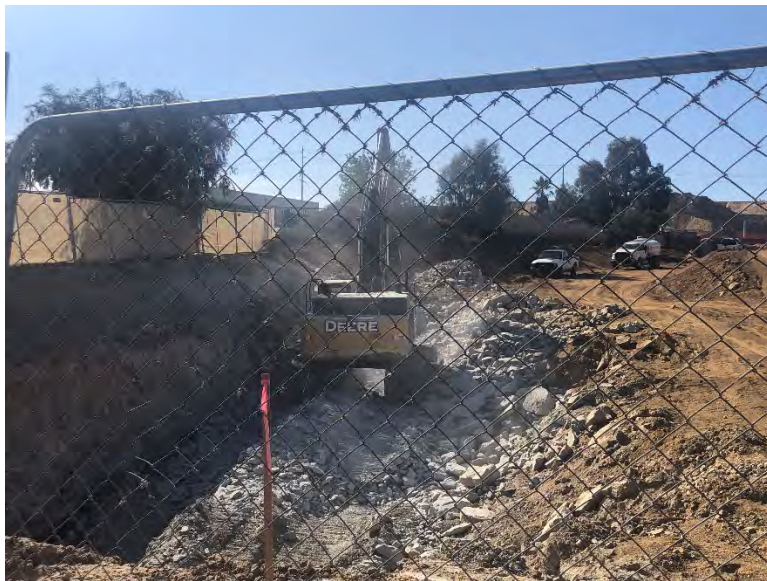
Photo 3: Southeast corner of Subject Construction
