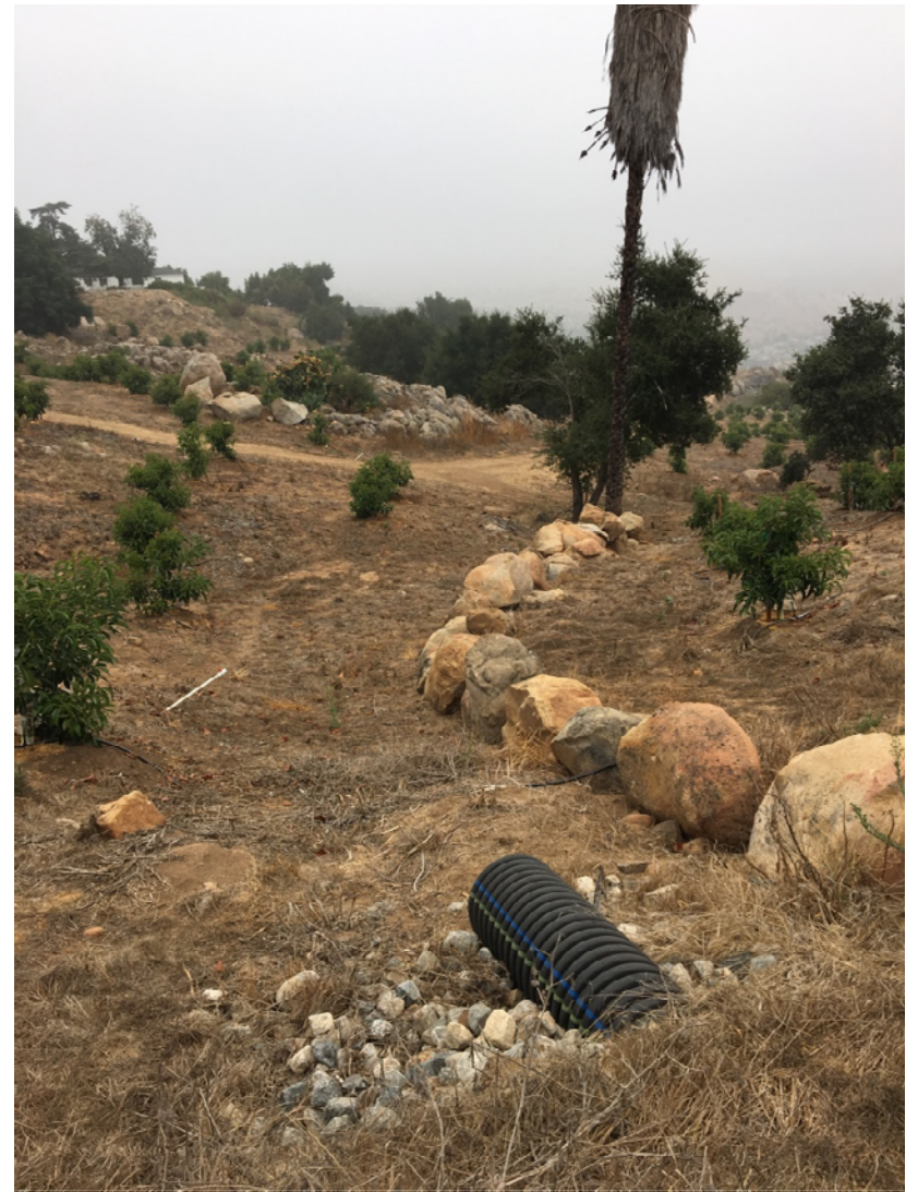
Photograph 6: Facing downstream at Feature 2 from the culvert depicted in photograph 5.
