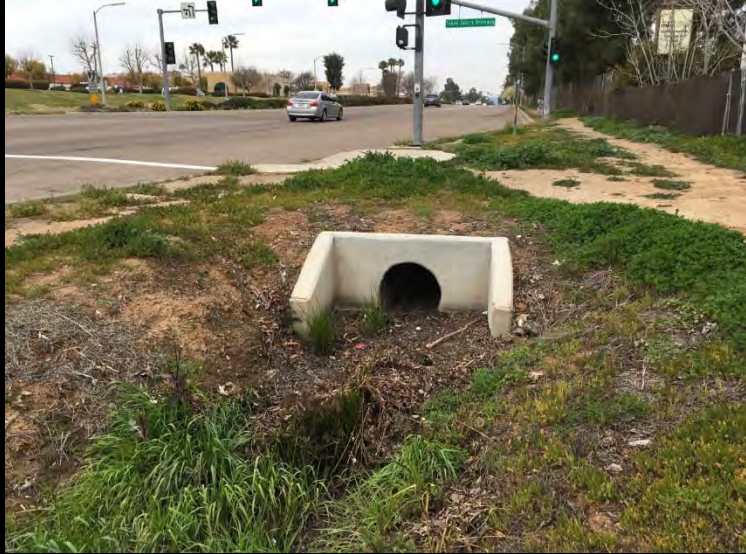
Representative Photograph 2. Facing N. Outfall at upstream end of channel.
