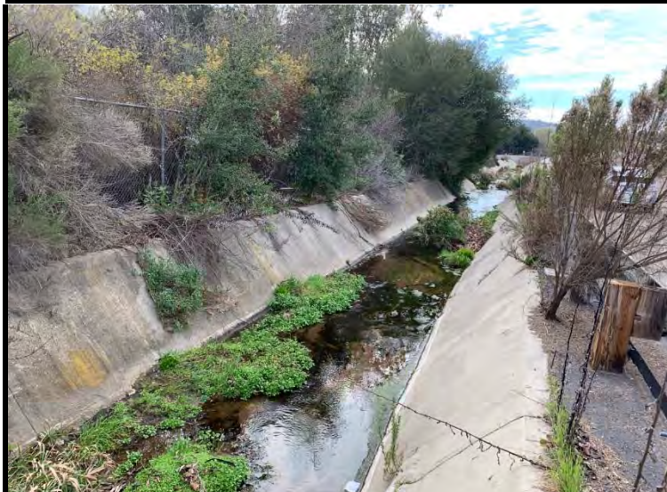
Representative Photograph 1. Facing NW. Concrete drainage channel
