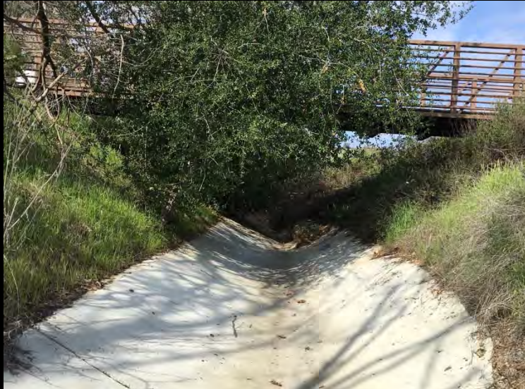
Representative Photograph 2. Facing NW. Concrete channel at upstream end as it flows under a pedestrian bridge crossing.
