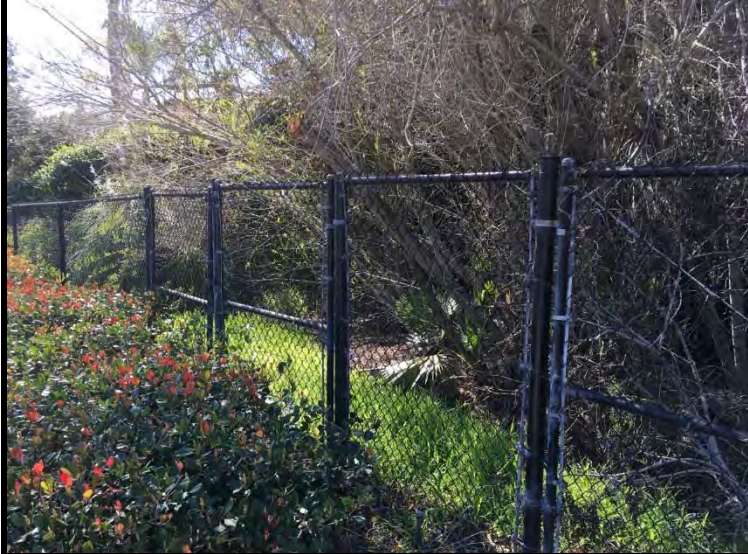
Representative Photograph 2. Facing SE. Fence surrounding basin
