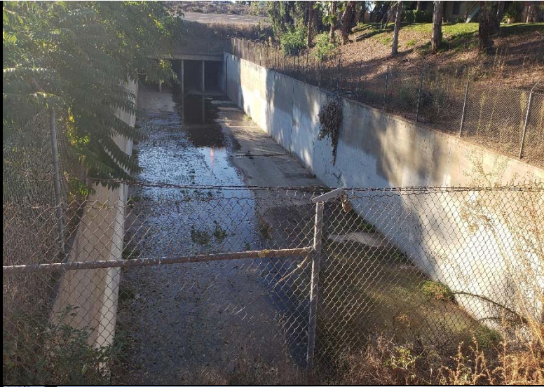
Representative photo of the southern section of the maintenance site, a concrete-lined channel.
