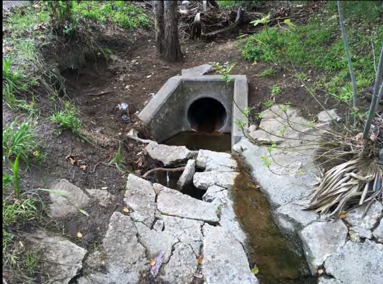
Representative Photograph 3. Facing S. Inlet at downstream end of channel
