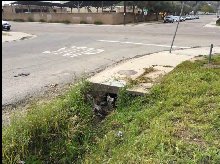
Representative Photograph 2. Facing W. Inlet at west end of channel
