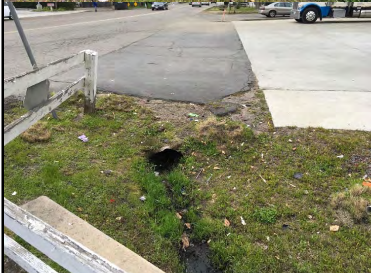
Representative Photograph 2. Facing W. Inlet
