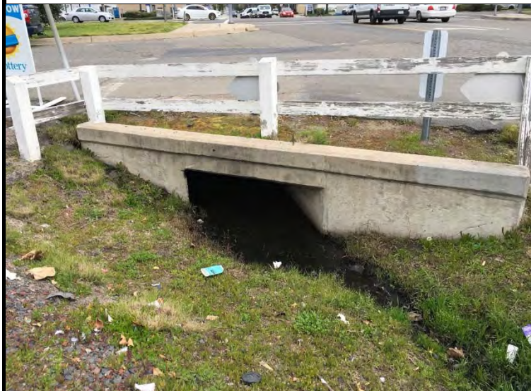
Representative Photograph 1. Facing E. Culvert
