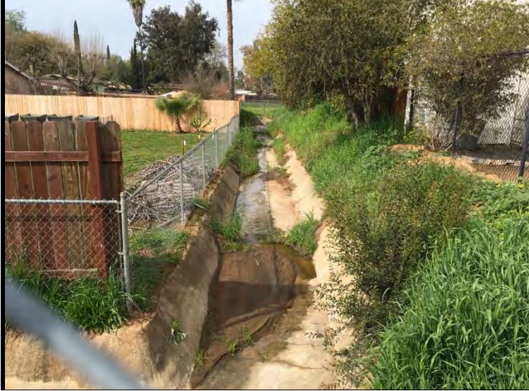
Representative Photograph 2. Facing W. Concrete-lined channel
