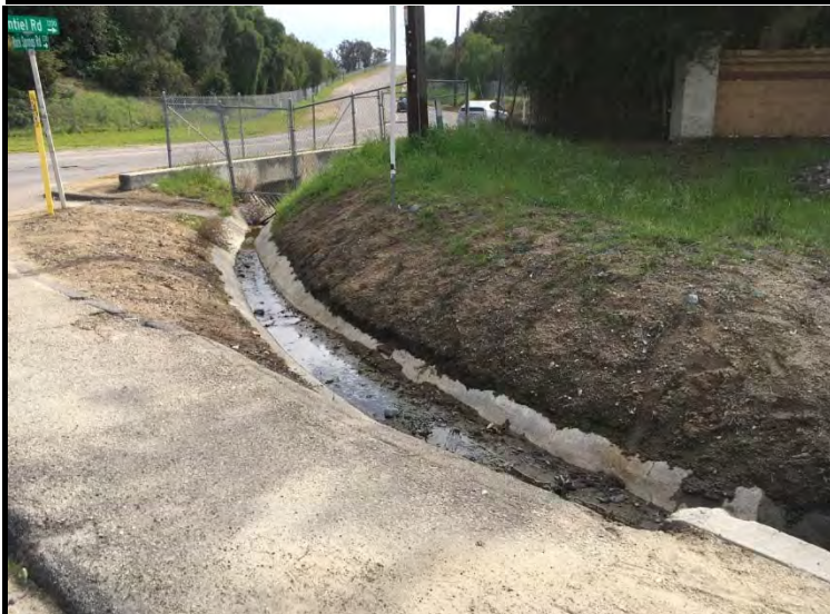
Representative Photograph 1. Facing E. Concrete-lined channel at downstream end
