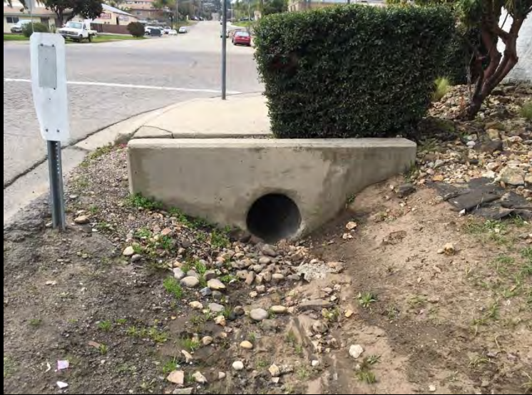
Representative Photograph 2. Facing W. Outlet
