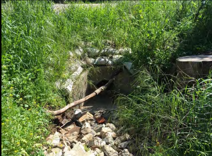
Representative Photograph 3. Facing E. Culvert under Bear Valley Road
