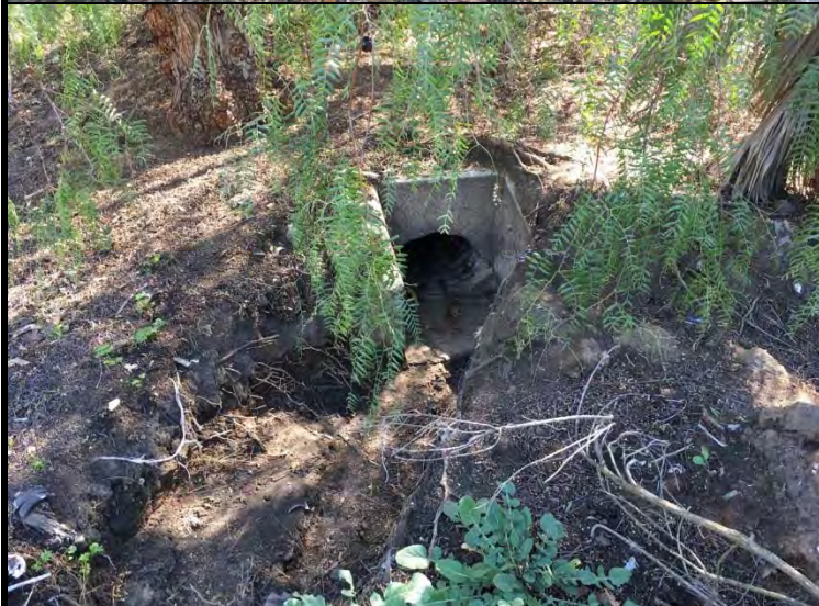
Representative Photograph 3. Facing E. Outfall
