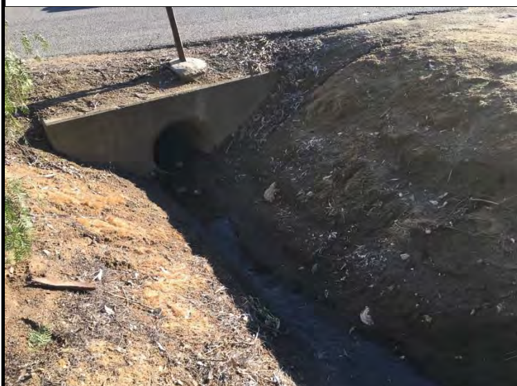
Representative Photograph 1. Facing S. Unvegetated channel and inlet
