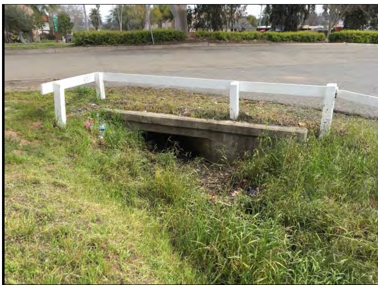
Representative Photograph 3. Facing E. Culvert at east end of channel
