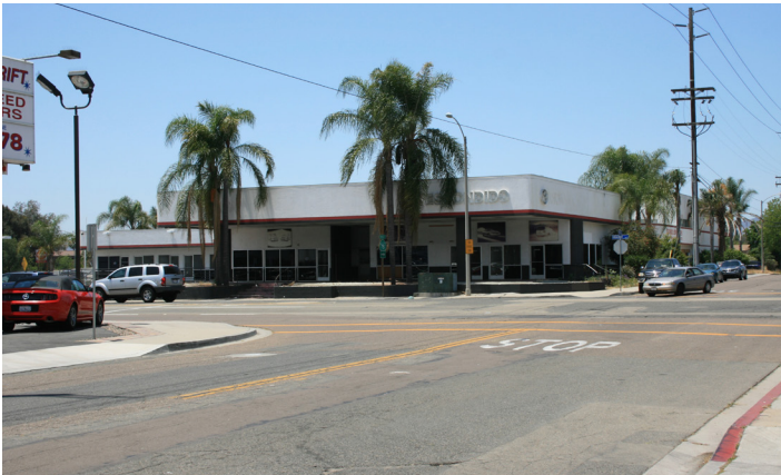
3 Candidate Key View #3: View from Lincoln Avenue looking west
