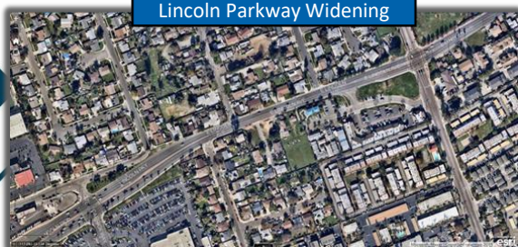
Lincoln Parkway Widening
