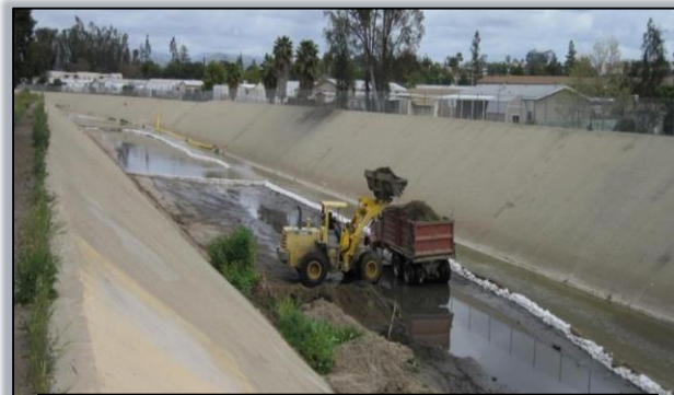
Permitted Channel Maintenance & Mitigation
