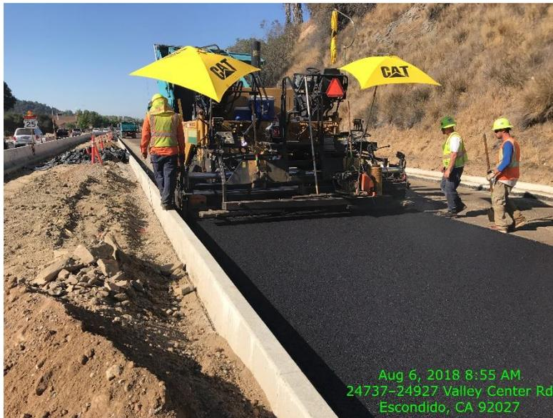
*Figure 3. Asphalt Base Pave along the West-side of the Project*
