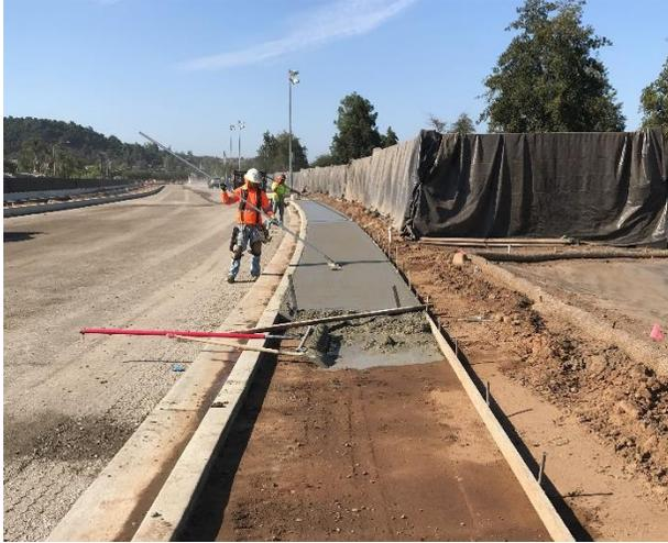
*Figure 1. Placement of Sidewalk Along West-side of Valley Parkway*
