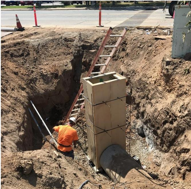
*Figure 2. Construction of Catch Basin Structure*
