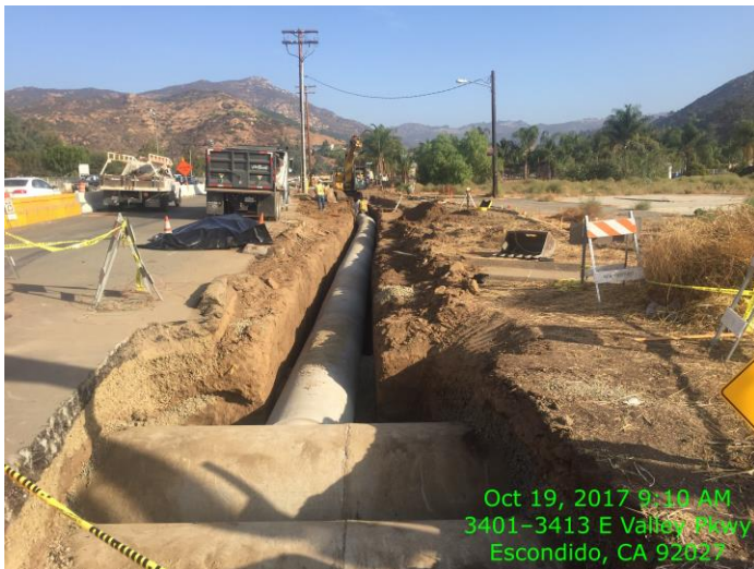
Storm Drain Installation
