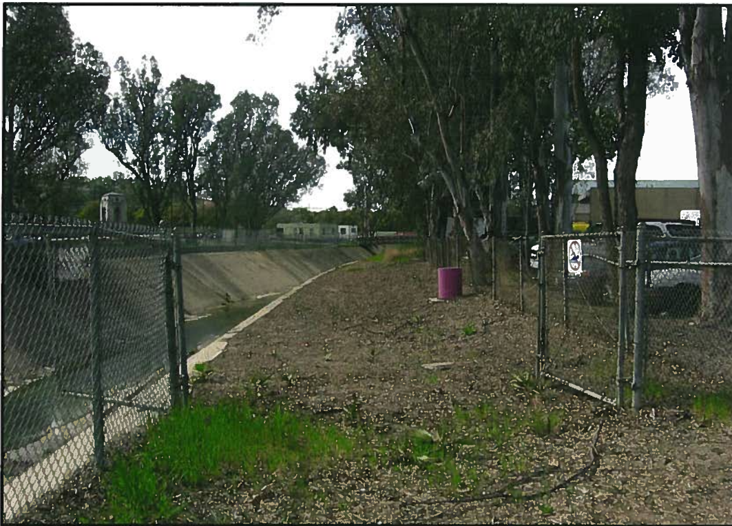
Figure 4 Looking west along north side of channel from Quince Street entrance.
