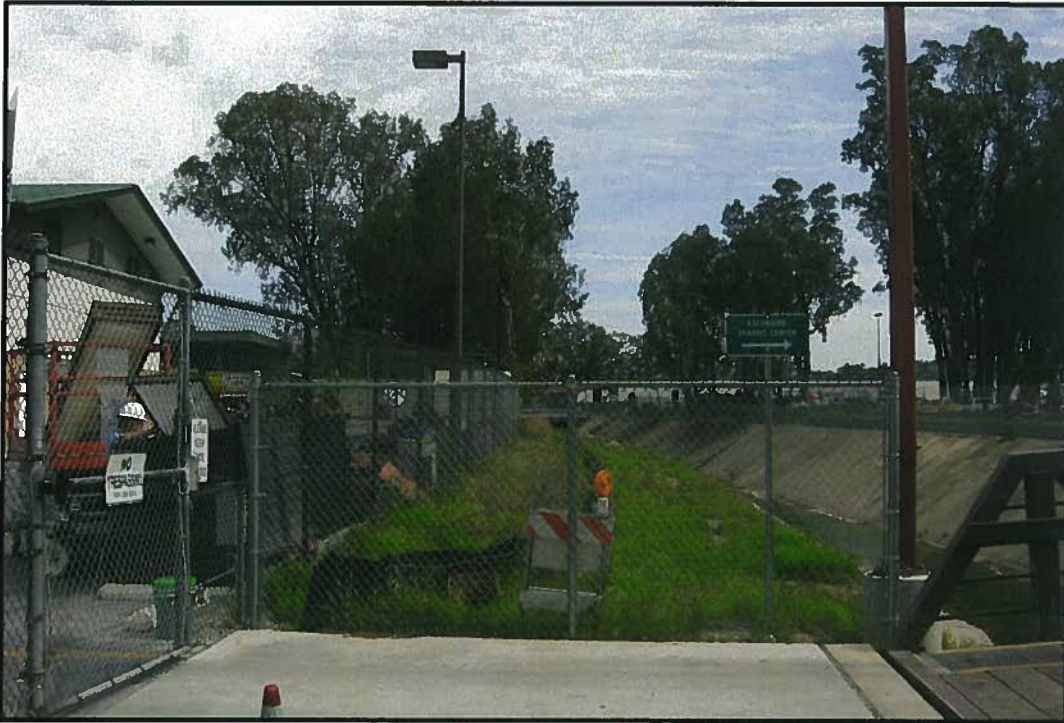
Figure 3 Looking east along north side of channel from Bridge towards Quince St.
