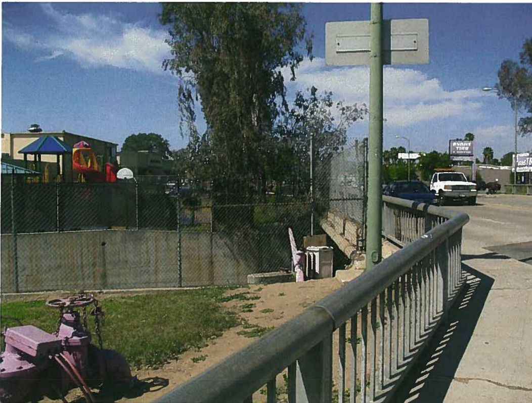
Figure 18 Road narrows at Escondido Creek
