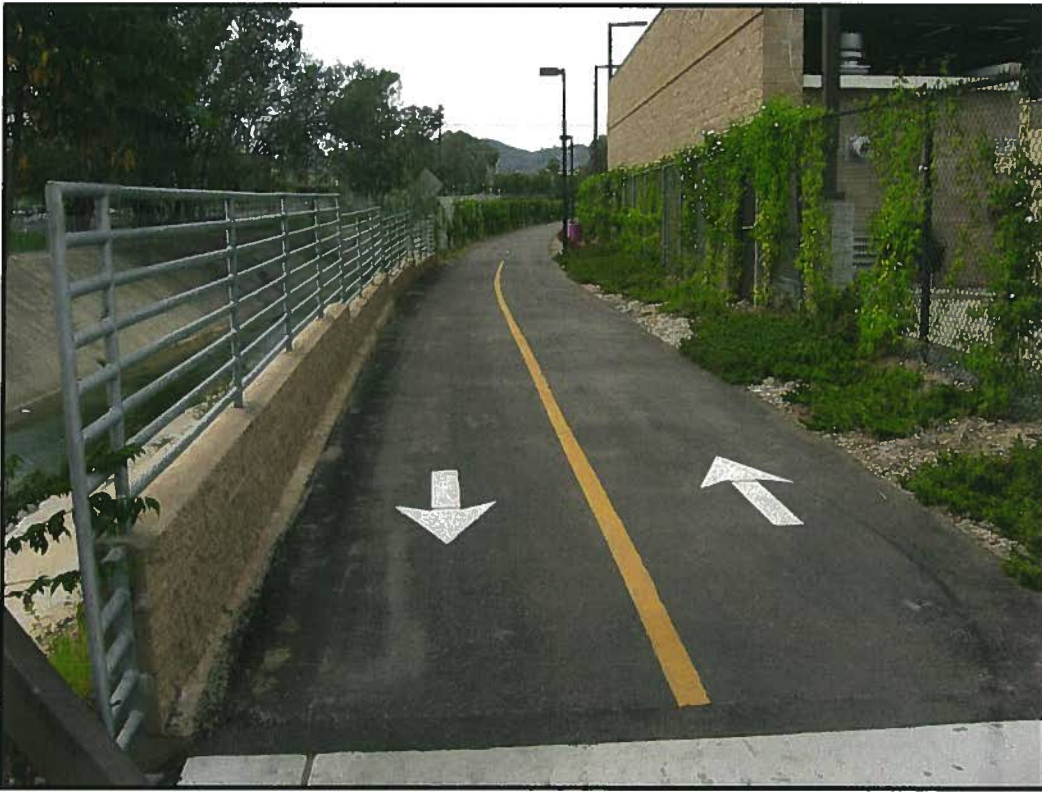
Figure 1 Looking west at Inland Rail Trail, north side of channel
