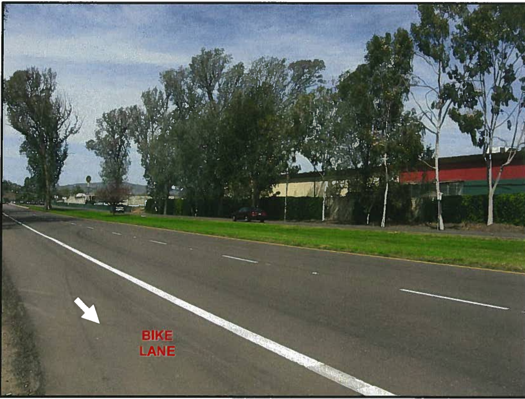
Figure 13 Looking north along Centre City Parkway at southbound lanes
