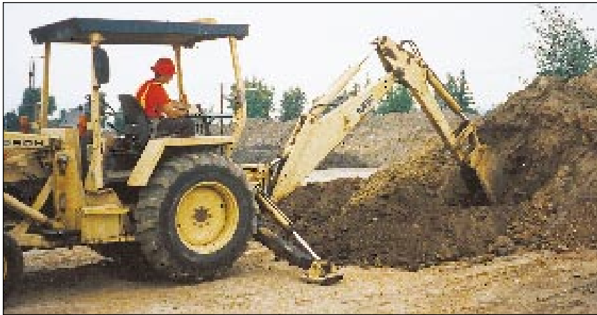
The backhoe operator practices stick control on a spoil pile.
