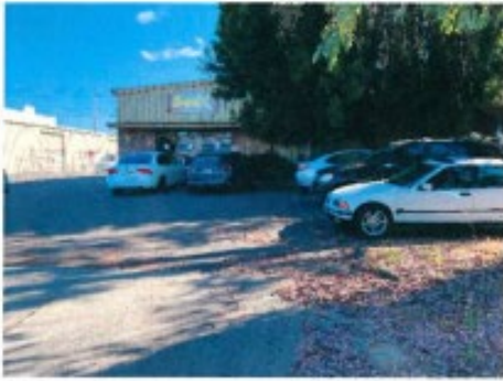
Figure 1 Looking toward building from the street.
