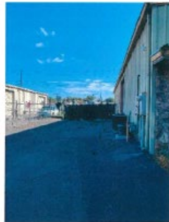
Figure 5 Looking toward rear yard at side of bldg.
